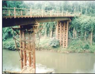
KAMUSIE-PANAKAWA- HAIVARO BRIDGE LINK
