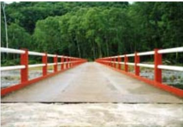
BRIDGE IN WEST NEW BRITAIN
